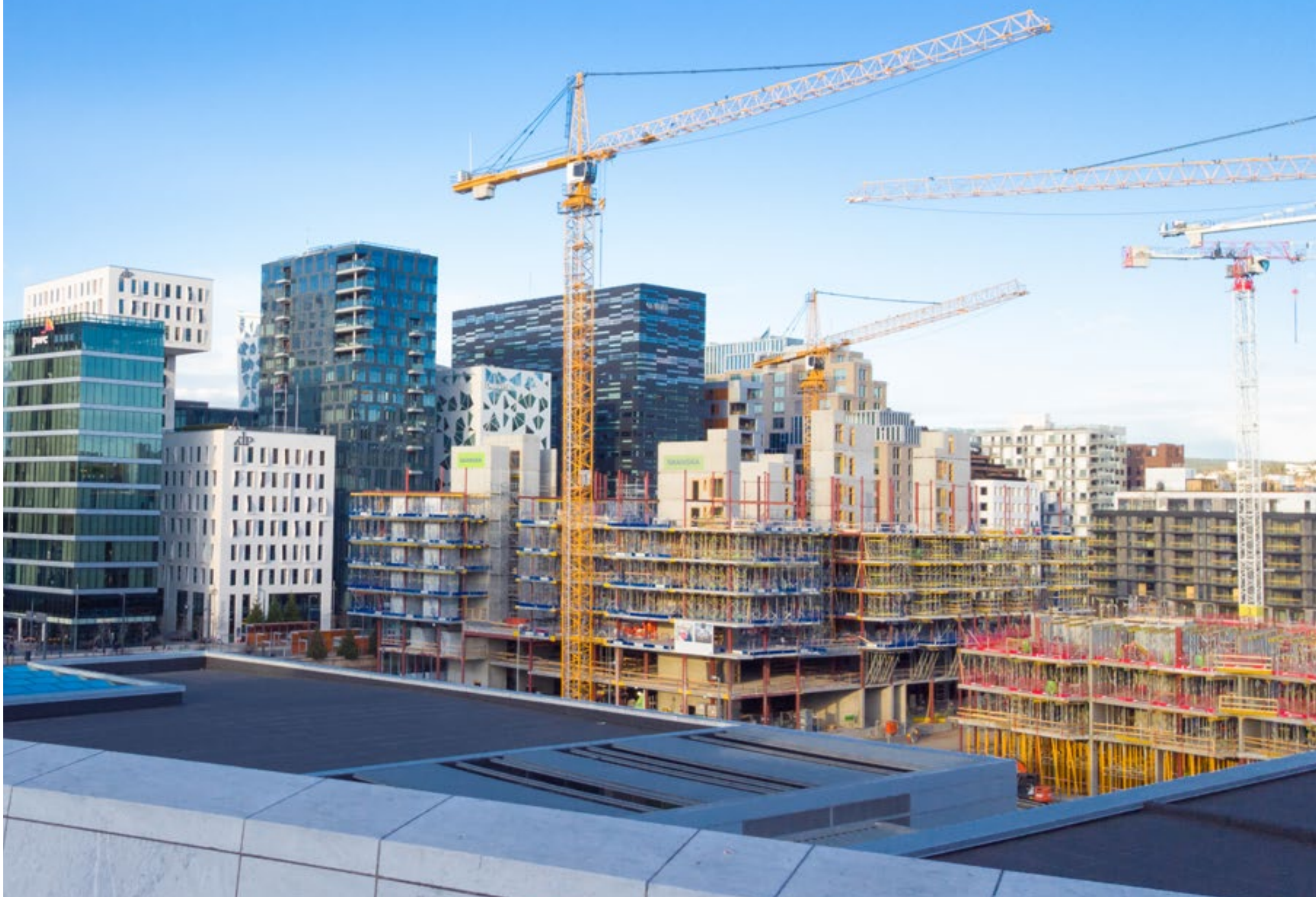
CONSTRUCTION IN OSLO, NORWAY
